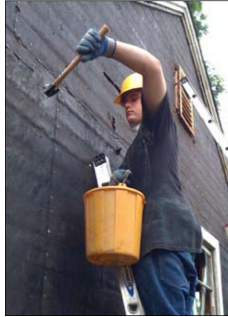
Kris Houser from St. Luke's removes old siding
